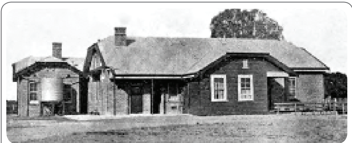
The 1936 Bush Nursing Hospital which contained 6 ward beds, 4 emergency beds, an x-ray plant and operating theatre. The building cost approximately 4,000 pounds to build.
