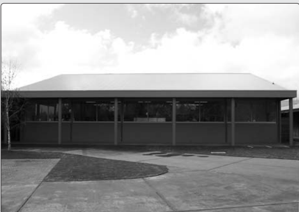
Benalla Health's new kitchen
